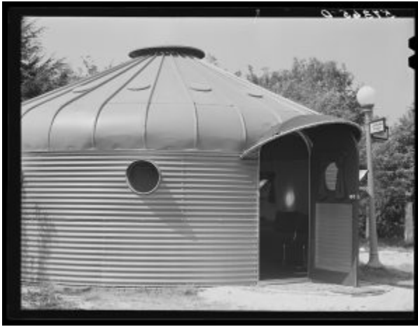
Buckminster Fuller, 'Dymaxion House,' 1941, Metal, Built for U.S. Farm and Securities Administration
